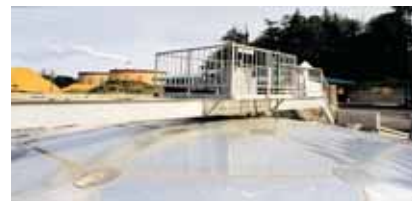
BST thickener with basin cover constructed beneath mechanism support bridge
