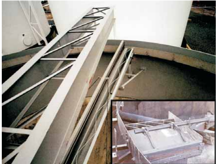
Optional full radius skimmer and trough (Inset) Standard skimmer and scum box
