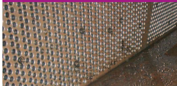
Tube condition with debris filter
