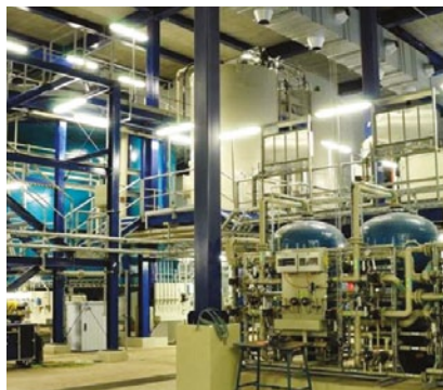
View from ground floor
