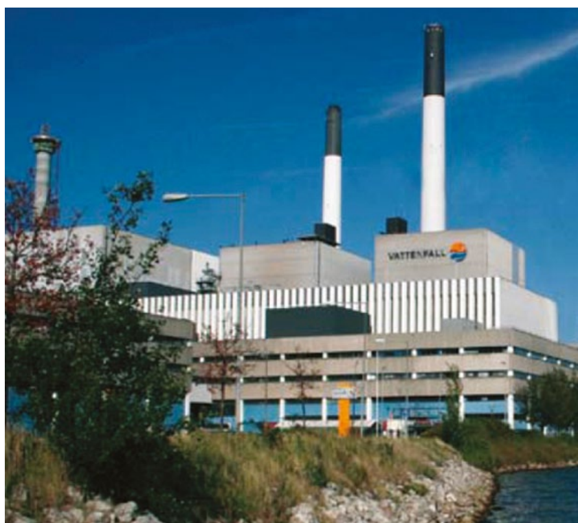
Coal and biomass fired power plant Amager II / Denmark
