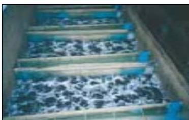
*These photos show the retrofitting of an 11' x 30' filter cell with Flexscour® underdrain components. This is one of sixteen cells refurbished with the Flexscour® system at the Medicine Hat, Alberta municipal waterworks. Average installation time for a four man crew was 41/2 days per cell, including demolition.*
