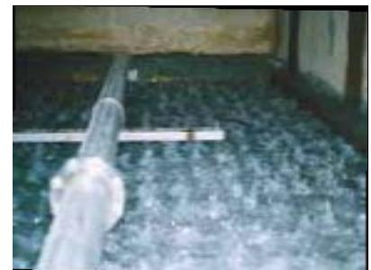
Photo above: Illustrates the uniformity of the air distribution in this new Flexscour® underdrain installation at the Medicine Hat, Alberta WTP; the photo was taken less than two seconds after the start of the air scour.
