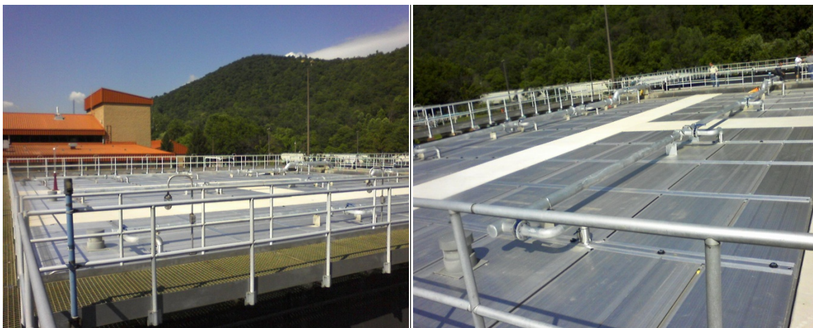
Figure 1. Bellefonte WWTP M-T.A.D. ™ Facility
