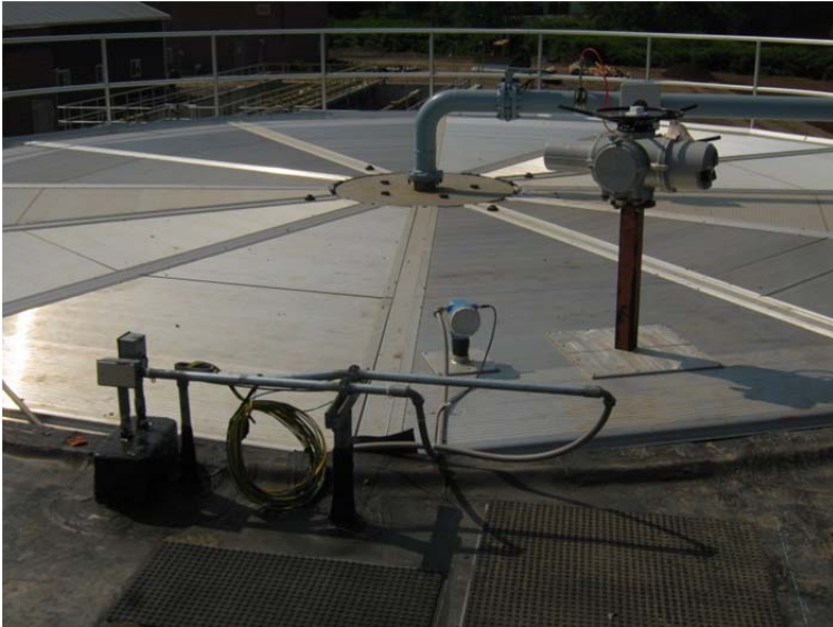
Airbeam Cover Aerobic Digestion System
