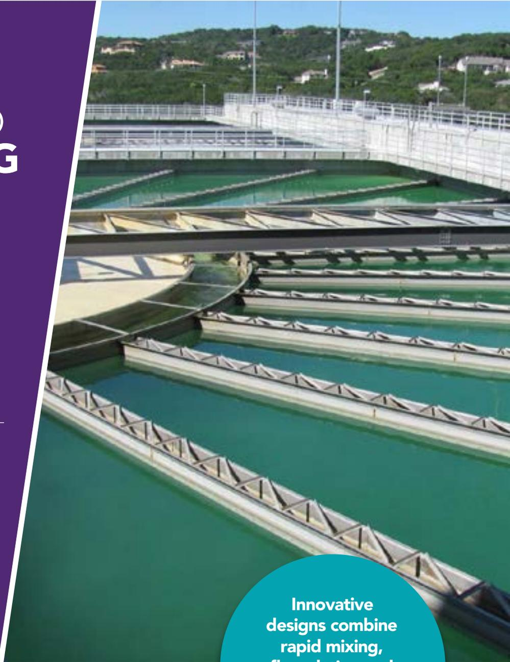
**Innovative designs combine rapid mixing, flocculation and clarification in a single tank for efficiency & land savings!**
