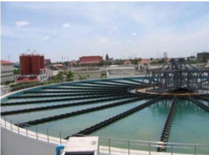
**TOP LEFT:** 42ft diameter HRB Type Reactor Clarifier™ Unit with steel launders, in Florida, USA
