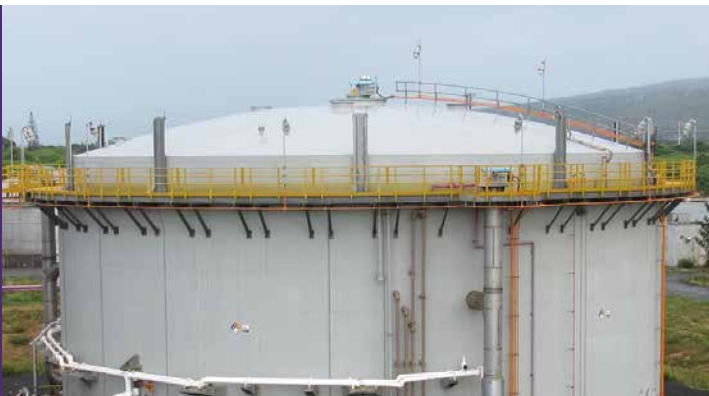
Honouliuli WWTP, HI (90' G2VL): Gasholder Steel Cover
