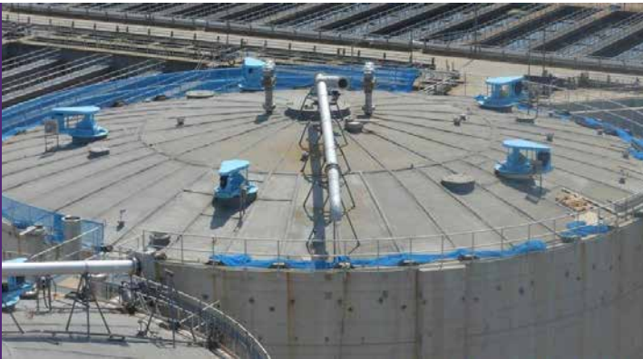
DC WASA, DC (98.5' F2) : Fixed Steel Cover
