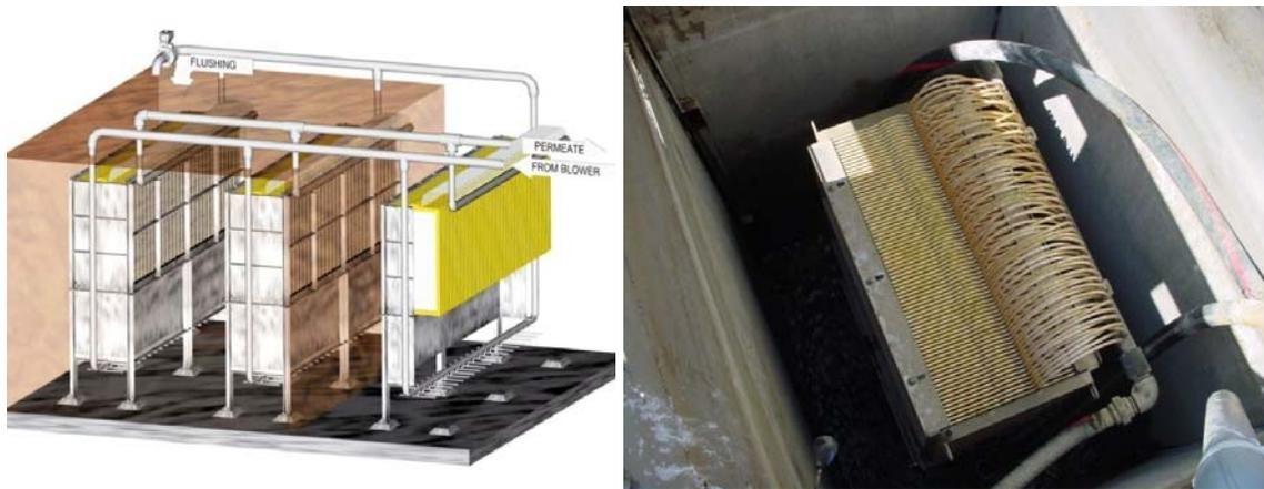
Wastewater is physically filtered out a submerged membrane unit (SMU) and is called permeate. This is accomplished because a coarse bubble diffuser located at the bottom of the unit creates a vacuum pressure gradient allowing for the wastewater to be filtered out of the sludge. The solids are left in the thickening tank while permeate is pumped via a progressive cavity or centrifugal pump to the head works of the plant or to disinfection. The diffuser also scours the membrane
