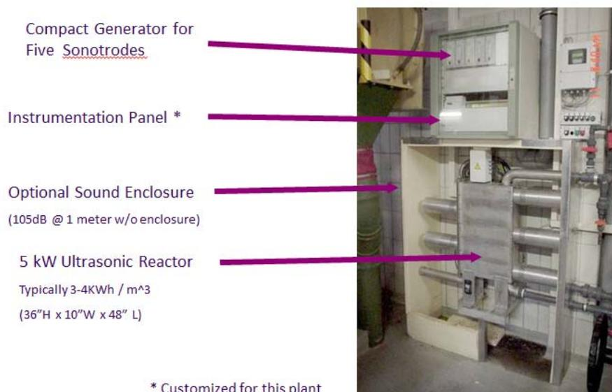
**Figure 2 - Ultrasonic Reactor**
