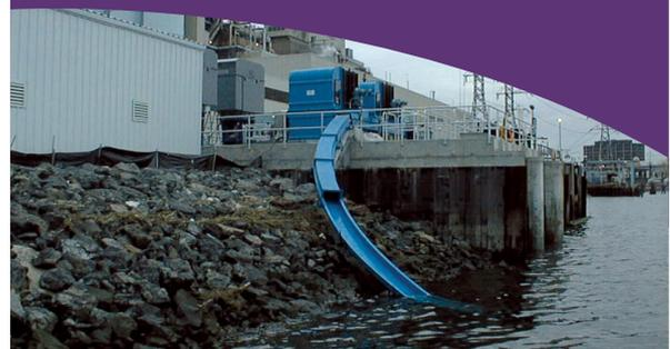
Traveling band screen with S.I.M.P.L.E.<sup>®</sup> fish recovery and return system
