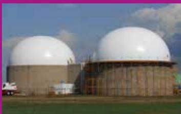
The  $\frac{3}{4}$  sphere can increase capacity for gas storage with a minimal impact on footprint. Usually designed for slab mounted options, the  $\frac{3}{4}$  sphere can be installed on a tank if the layout permits it.
