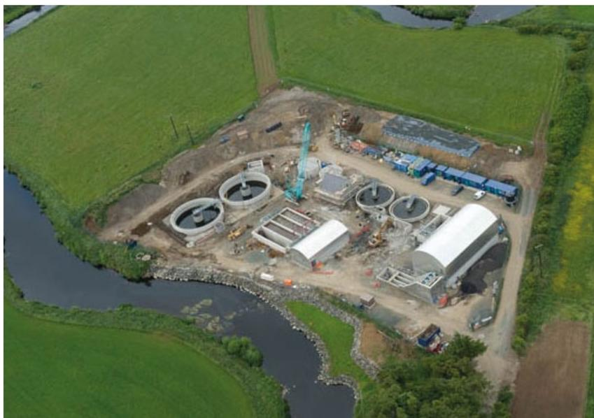
facility for treatment before being discharged to the River Bush. The wastewater treatment facility at Portballintrae was then refurbished to provide additional storage capacity for stormwater.
